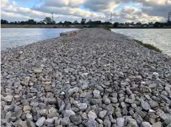
Ham Pier 27 dyke wall improvements
