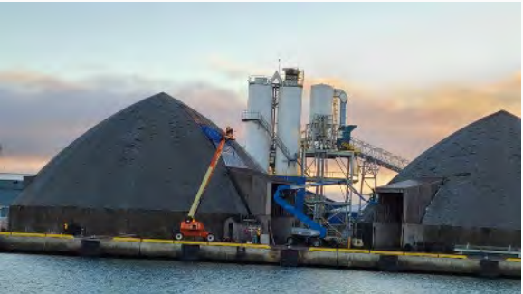
Oshawa dome roof replacement
