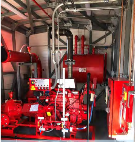
450 Sherman fire upgrades
