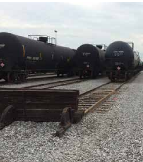
Pier 22 rail reconstruction
