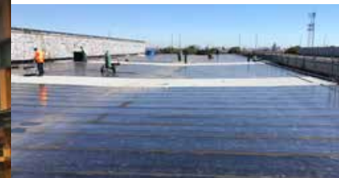
1632 Burlington St. partial roof replacement
