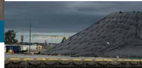
Eastport dock fenders, ladders, wheel guards
