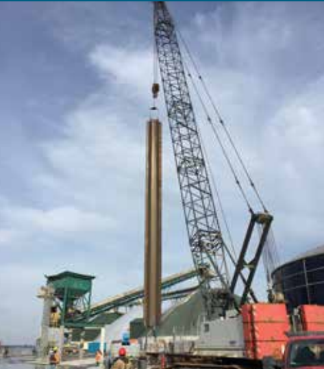
Pier 12 west wharf reconstruction – phase 1
