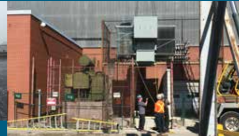
1632 Burlington St. transformer replacement
