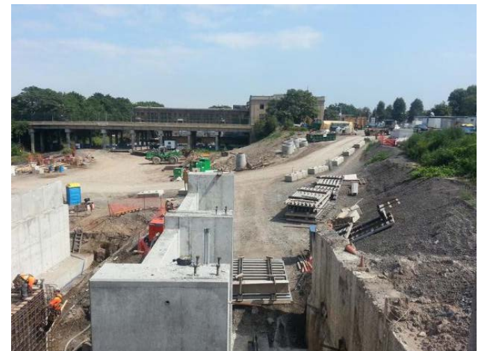
James Street North GO Station Under Construction
